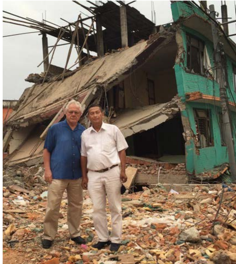
■ The city after an earthquake
