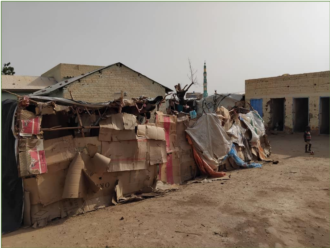
Emerging structures in towns due to severe economic realities.
